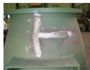
Crack fully repaired
