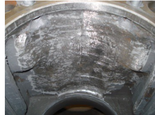
cavitation grinded back to original
