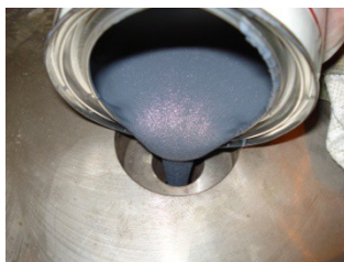
Grouting from a can
