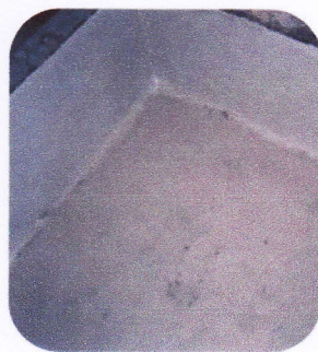
Priming of storage tanks
