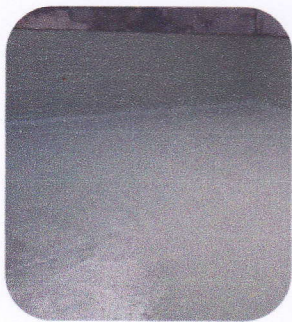
Priming of concrete bund areas
