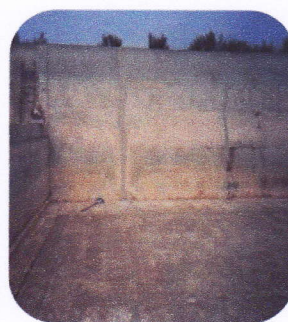
Sealing porous concrete surfaces
